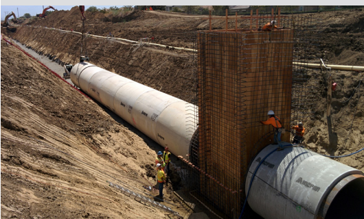
ABOVE: Segment 2 construction
