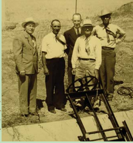
The first delivery of water from the Contra Costa Canal was made in 1940.
