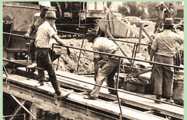
Construction of the 48 - mile Contra Costa Canal took 11 years from 1937 to 1948.
