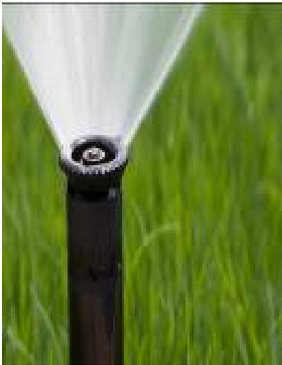
To reduce water running off your lawn and landscape, use the cycle and soak method to water. For standard pop-up spray sprinklers, set your timer to water for 4 to 6 minutes at 4:00 AM, 5:00AM and at 6:00AM. This will ensure the water soaks into the soil rather than running off. The watering days per week will vary depending on the weather. Generally in June and July lawns will need 3 to 4 days per week.
